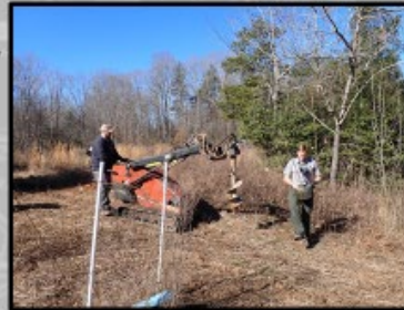
Engineering Tech Tim Taylor (l) and Ranger David Bolick (r) using auger to dig holes.
